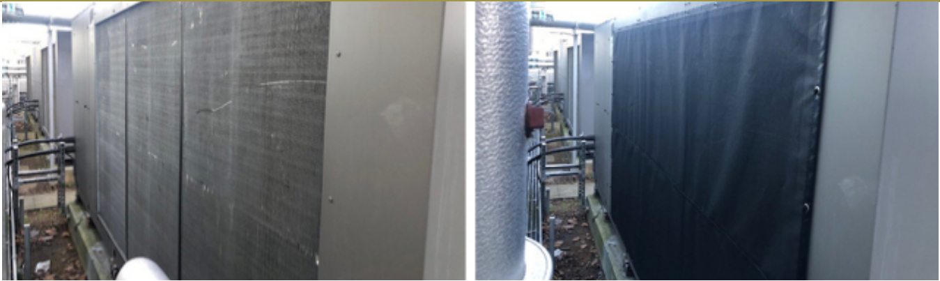
Example of a cooling unit before and after installing a Permatron PreVent® intake filter screen
