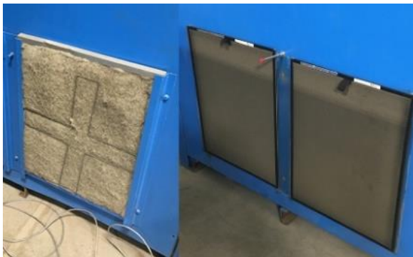
Compressor intakes protected by polyester media on the left-side and the PreVent® screens on the right.
